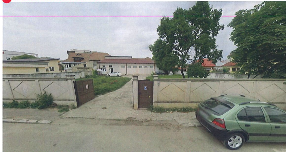
12. CONSTRUCTIA CARE A GENERAT PUZ, CONSTRUCTII EXISTENTE ANEXE
